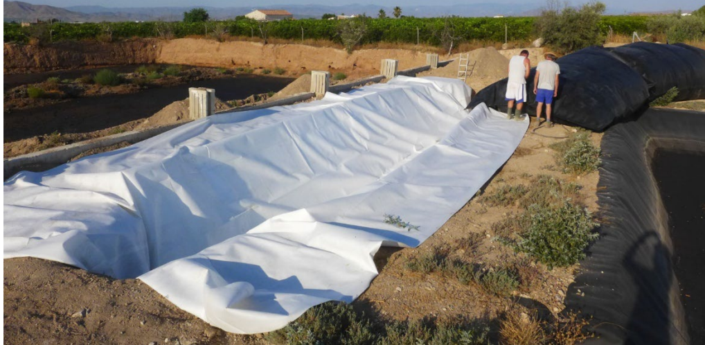
Geomembrane inflated in the trench
